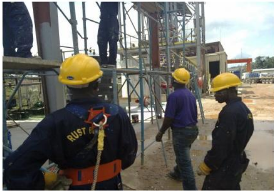
RUST BULLET APPLICATION ON CYNIDE STRUCTURE~EXTERNAL REAGENT AREA AT GOLDFIELDS GHANA LTD, TARKWA
