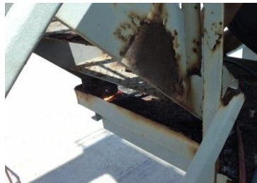
Corrosion on crane
