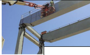
Spraying Rustbullet onto columns, using piston spray machine 2400psi.
