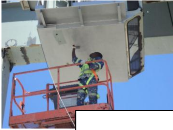
Rolling Rustbullet onto control cabin, using foam rollers
