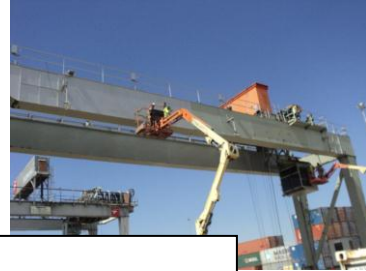
Spraying Rustbullet onto columns, using piston spray machine 2400psi.
