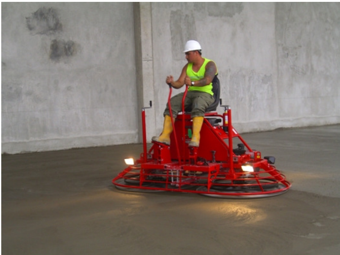
8) Panning of wet concrete floor using rider trowel
