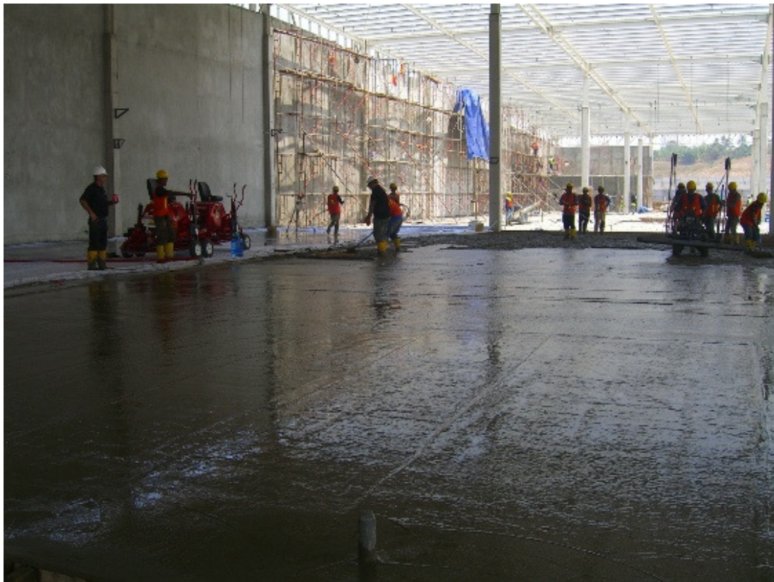
6) Waiting concrete to gain strength before trowelling
