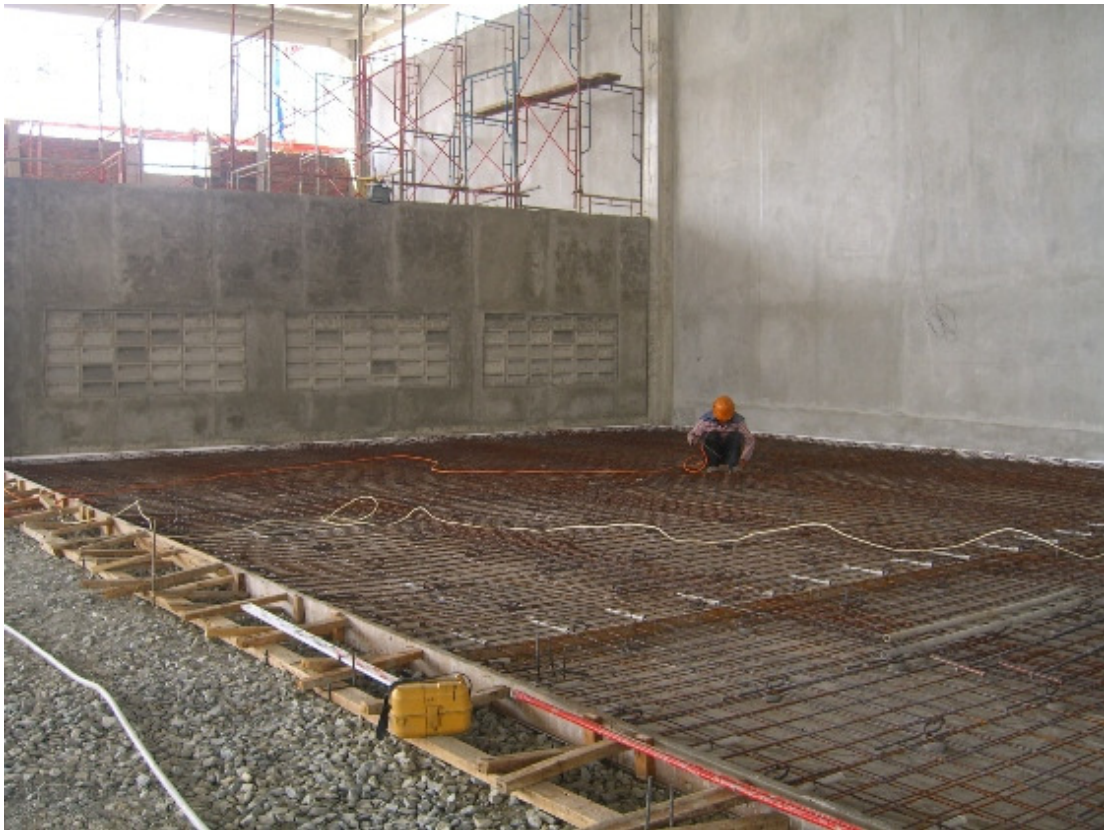
1) Preparation of rebar and formwork
