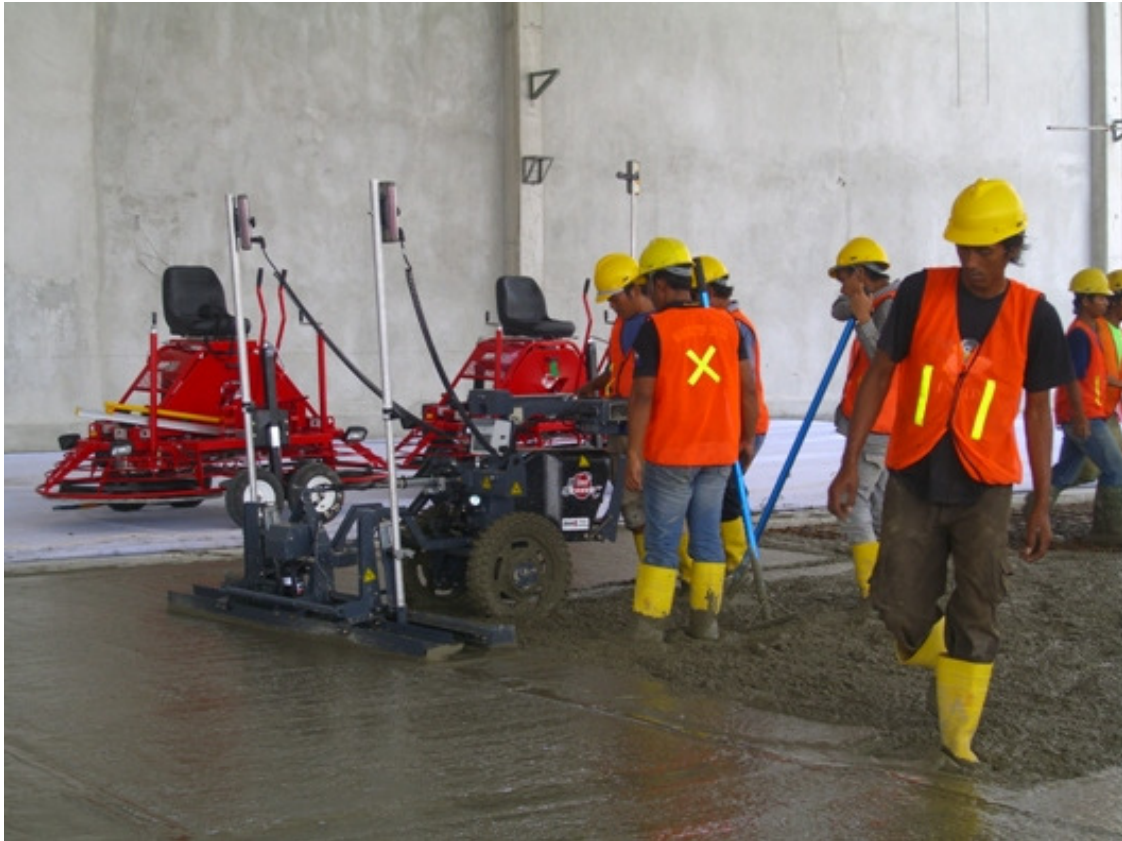
3) Leveling concrete using lazer screed
