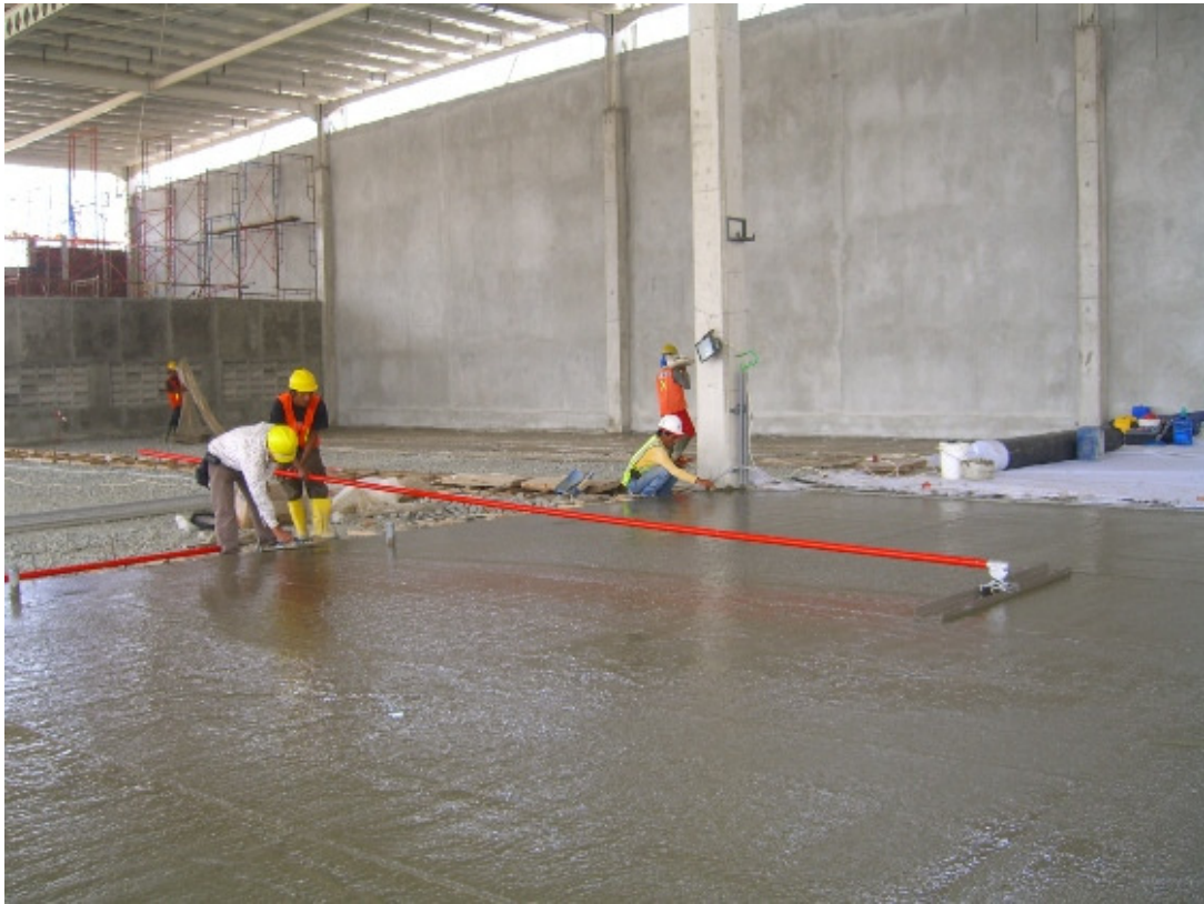
5) removing uneven areas using channel float
