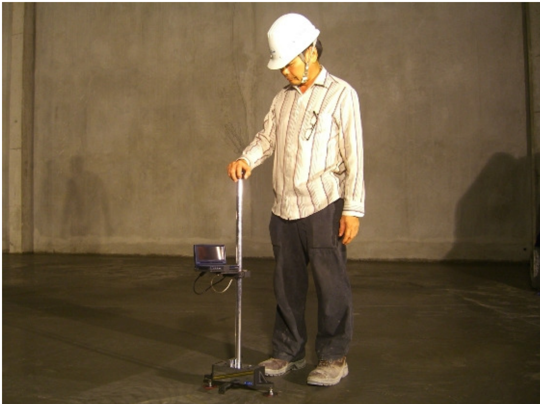
10) Floor profile measurement using Dipstick
