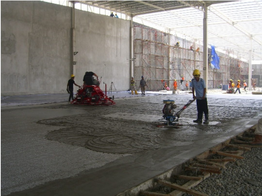
7) Trowelling using walk behind power trowel
