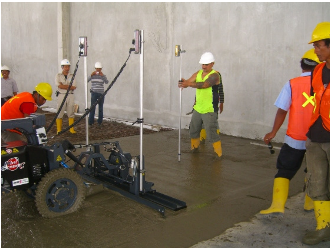
4) Checking wet concrete finish elevation using lazer level
