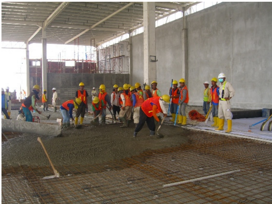
2) Pouring of wet concrete
