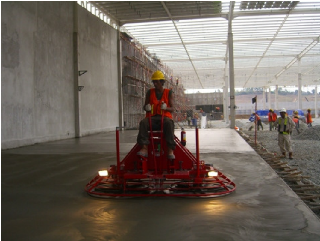
9) Trowelling using rider trowel to achieve flat surface
